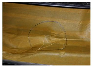
Within the marked circle, drill a hole for the start point of cutting.
