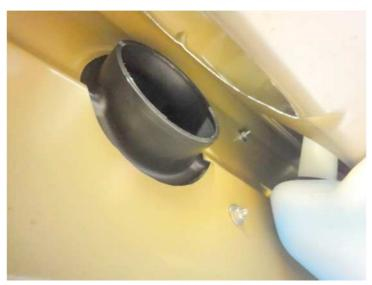
Tighten all the 4 screws at the bottom with nuts and washers from the inside.
